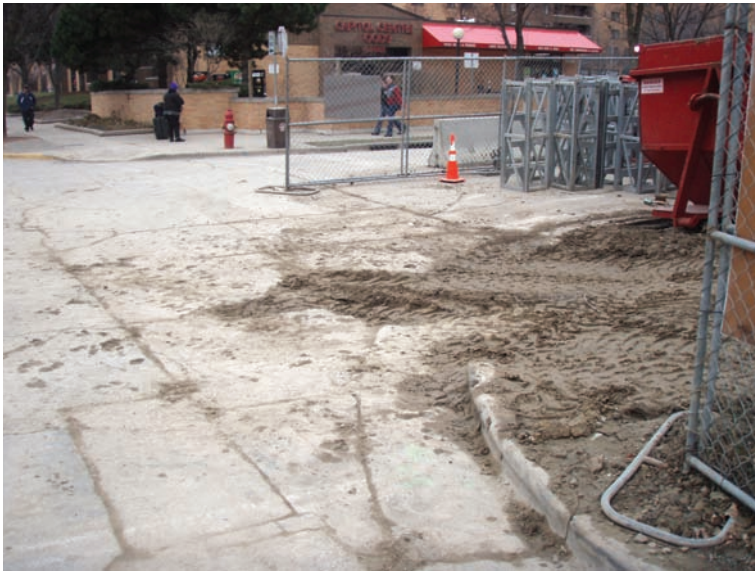
Figure 6.1. Sediment tracked onto street from equipment at a construction site in the Monona Bay watershed.
