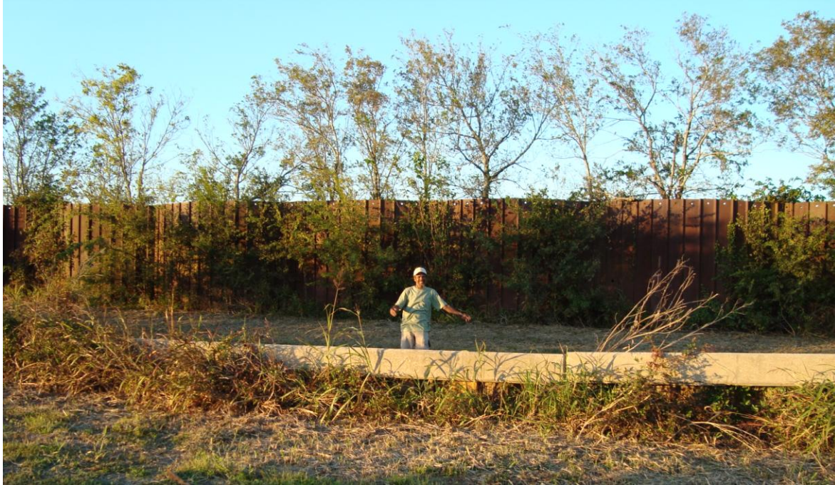
Figure 1-6: Lower Ninth resident John Taylor, next to the old Florida Avenue Floodwall (foreground), which was chest high in the mid-twentieth century, but the land has since subsided several feet. The current floodwall can be seen in the background. (Photo by Lauren Brown, November 2008.)
