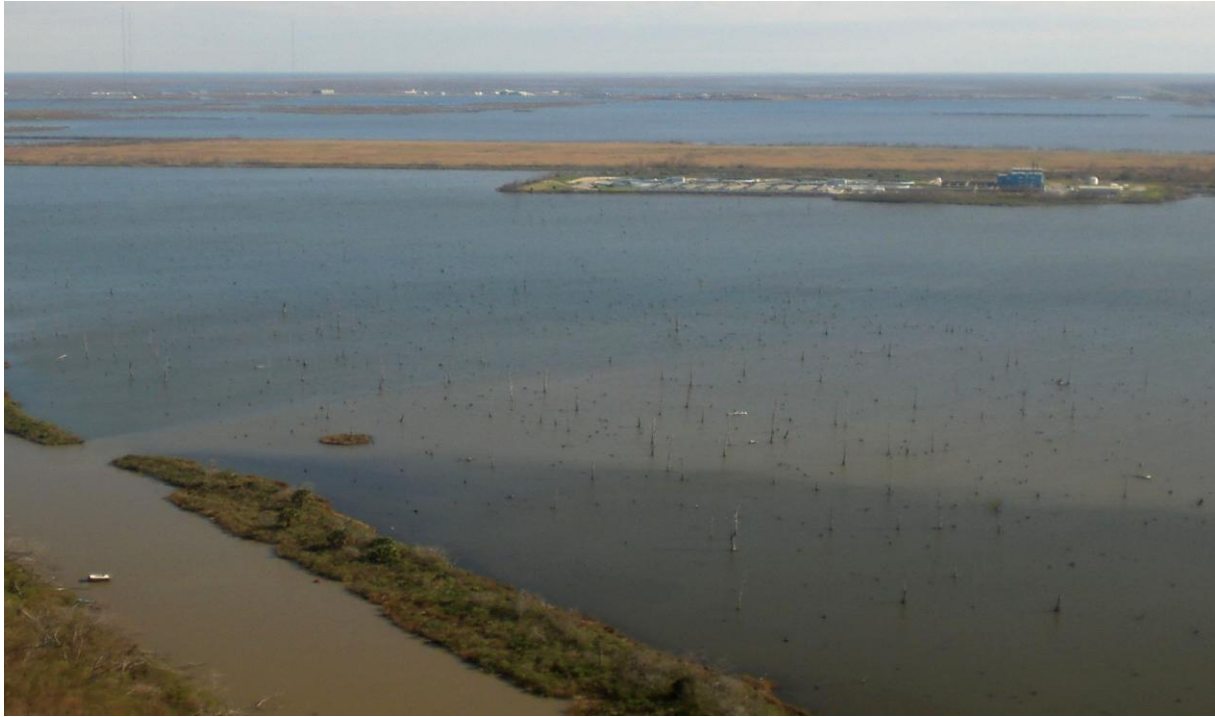
Figure 2-4: Pump Station 5 effluent entering the BBWT through the westernmost opening in the spoil bank. (Photo by Dan Cornelius, January 2008)
