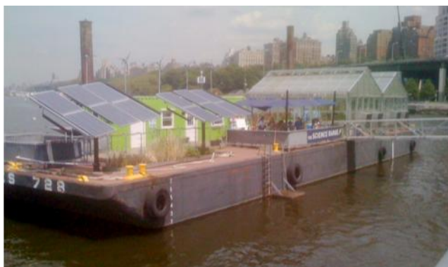
Figure 9-4: Hudson River Science Barge. The floating urban farm with wind turbines, solar panels, and greenhouses is docked to a pier in the Hudson River in August, 2008.
