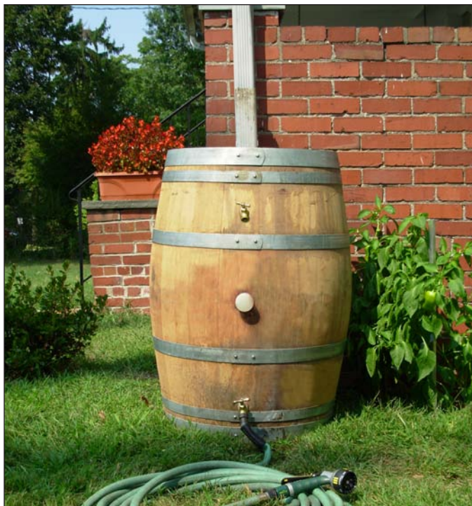
Figure 15.8 An example of a rain barrel. Source: Center For Watershed Protection, Urban Stormwater Retrofit Practices. http://www.cwp.org/PublicationStore/USRM.htm#usrm3
