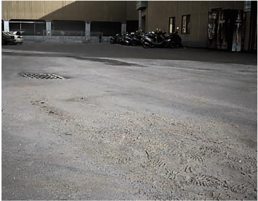
Figure 4.13. Sand used for traction in the winter accumulating near a stormsewer inlet at Camp Randall. To avoid sedimentation of stormsewers and lakes, an increased budget for street sweeping and hand sweeping of the sand must be provided to the numerous campus departments that have this task.
