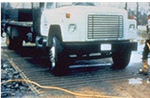
Figure 4.4. Example of a rubberized washing pad in action. Picture taken from http://www.epa.gov/owow/images/NonPtPics/14.GIF .
