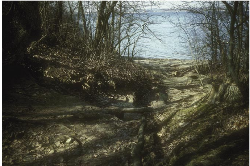
Figure 1.4. Gully erosion at Angler's Cove below a stormsewer outfall.
