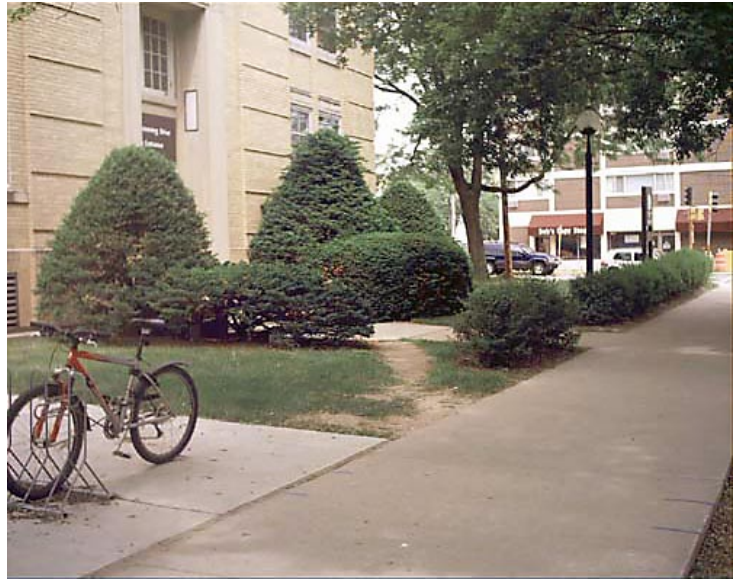
Figure 4.11. Example of a dirt convenience path at Computer Aided Engineering Building causing compaction and erosion problems. This would be an excellent location to add more bushes or a chain link fence located far enough back not to hinder snow removal.
